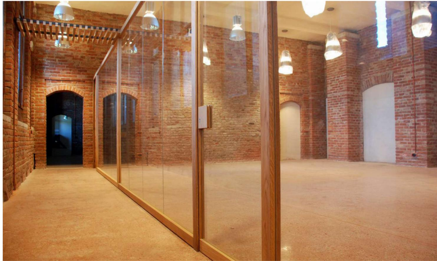
*The NORDWOOD system does not include upper or lateral adjustment panels. Each component is custom-made to meet the specific requirements of the project site. The single-glass configuration allows for the optional integration of a shading system consisting of adjustable wooden slats, maintaining the same overall dimensions while ensuring enhanced privacy for the spaces.*
